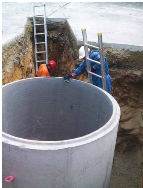
INFRASTRUCTURE WORKS: Underground tank to filter contaminants at the Council's Cleary's Gates Depot.
